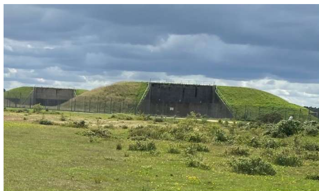
GREENHAM COMMON SILO
